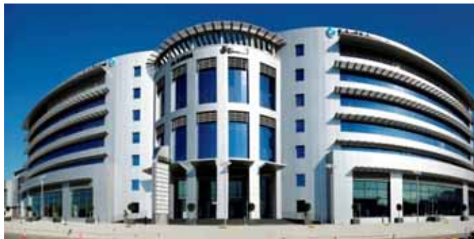
TAKAMUL CUC at Al-Rawaq Building Qurum
